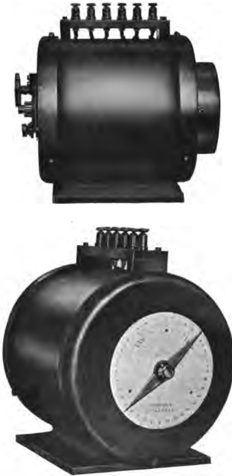
FIG. 10.—Drysdale Phase Shifting Transformer as made by Mr. H. Tinsley.
